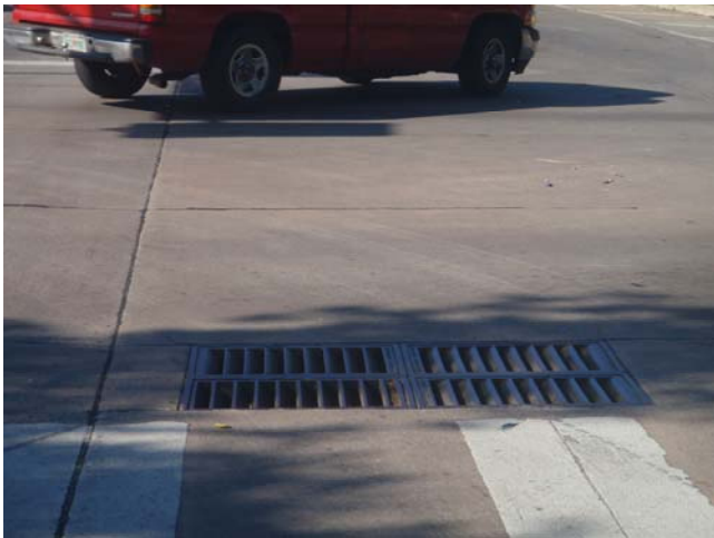
Above: Berry southbound, turn lane onto Boyd: Parallel Grate
